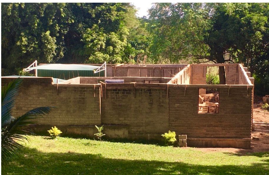
Figure 4: Newly developed distillation equipment building at MMCT offices, Mulanje
